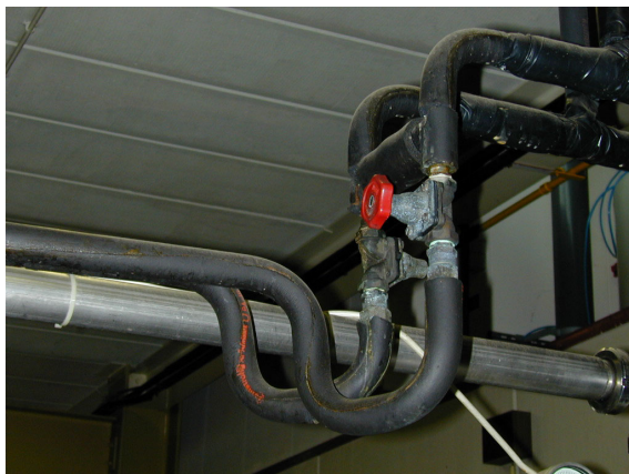
Figure 3.13 Incorrect installation of pipework: pipes can not be drained completely.
