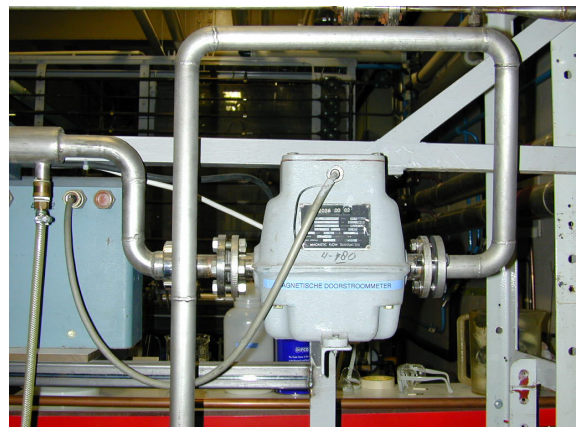
Figure 3.13 Incorrect installation of pipework: pipes can not be drained completely.
