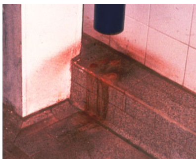
Figure 2.13 Sharp corners and build up of material on edges.
