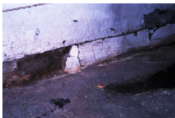
Figure 2.17 Damaged concrete allowing accumulation of product residues and microorganisms.
