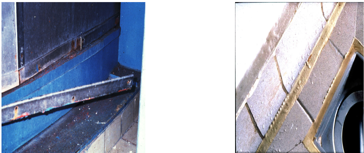
Figure 2.11 Sharp (left) and round (right) edges. Design of drain and floor material in right image is correct. Beware: seals must be maintained to prevent cracks and crevices.
