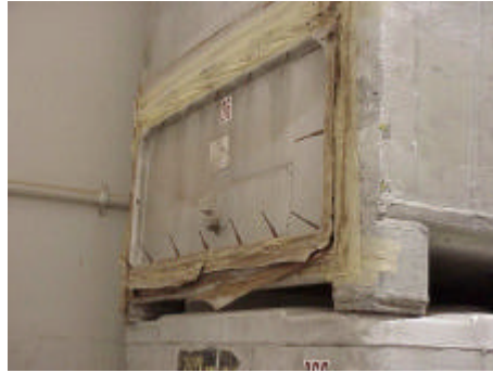
Figure 5.8 No good practice: 'temporary' fix with tape. Who knows where the pieces of the degrading material may end up.
