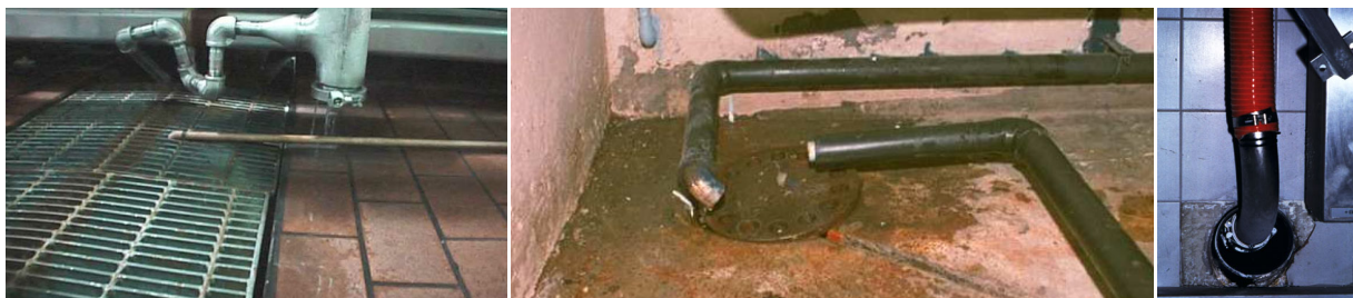
Figure 2.21 Pipes and equipment placed in and above gutter and drains. Difficult to open and clean.
